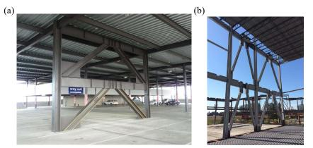
Figure 1. (a) Two-tiered eccentrically braced frame (MCEER report) [5]; b) Two-tiered eccentrically braced frame with replaceable links in Richmond B.C. [6].
